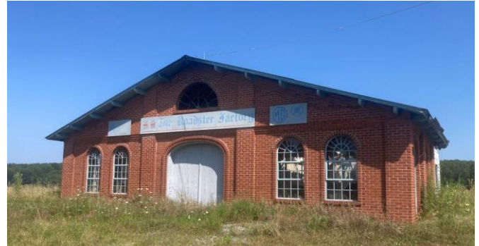
TRF6 – Front of what is left of the 'old' Roadster Factory
