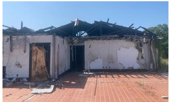
TRF7 – Rear of what is left of the 'old' Roadster Factory
